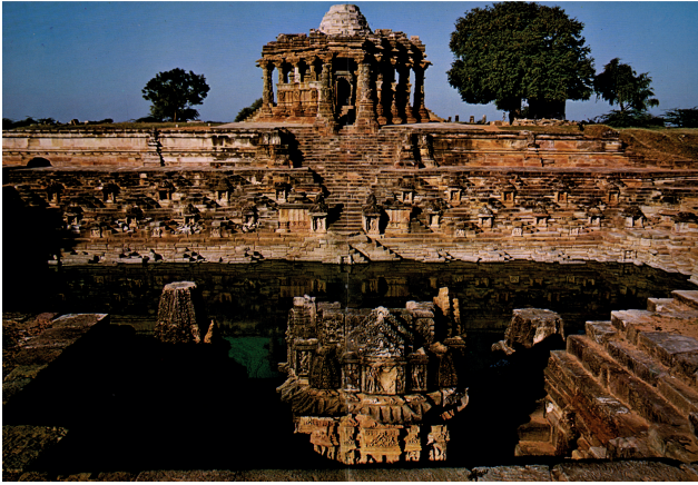
1026 a.d. Hindu temple at Modhera. The ruined stump of the sikara-mountain projects above the roof of the mandapa-portico.
